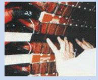
Iris Power Stator Slot Coupler Installation in a stator slot.
